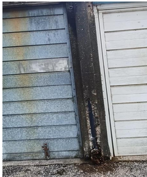
Frame detail with spalled concrete
